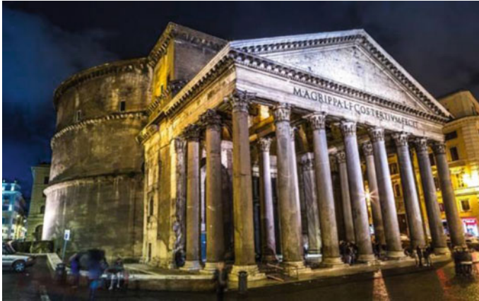
Fig. 1.5 Roman Pantheon —The first concrete building believed to be built in the world. The building has a largest unreinforced solid concrete dome (43.3 m diameter) built at that times. The building has sections large enough to keep the stress level in its different components sufficiently small to withstand the loads ( Source Internet)
