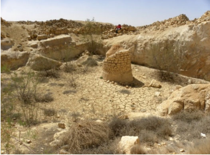
Fig. 1.2 Remains of a Nabataean cistern found north of southern Israel. Investigations discovered that it consists of hydraulic concrete made using lime as a cementitious material and were impervious enough to prevent the leakage of stored water into the soil ( Source Internet)
