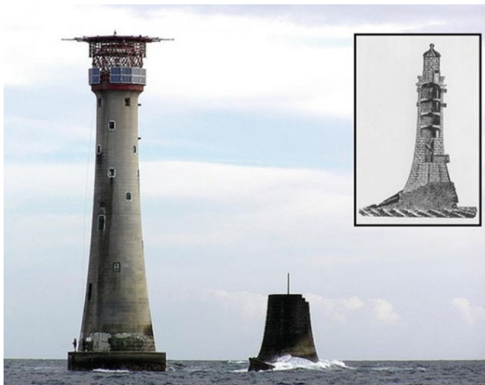
Fig. 1.6 Eddystone Lighthouse —The 18 m high lighthouse built by British John Smeaton (1759) on the Eddystone Rocks, about 14 km south of Rome Head, England (UK). The original lighthouse was built using the granite blocks joined together using ‘hydraulic lime’—a concrete that sets under the water, and the marble dowels. However, this structure was pulled down, except for its base and moved to Plymouth and then rebuilt it on a new base adjacent to the original location ( Inset the original Eddystone Lighthouse) ( Source Internet)
